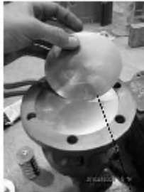
Remove & inspect diaphragms.
