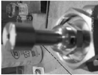
Inspect main valve.
