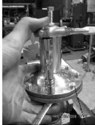
Remove spring case bolts.
